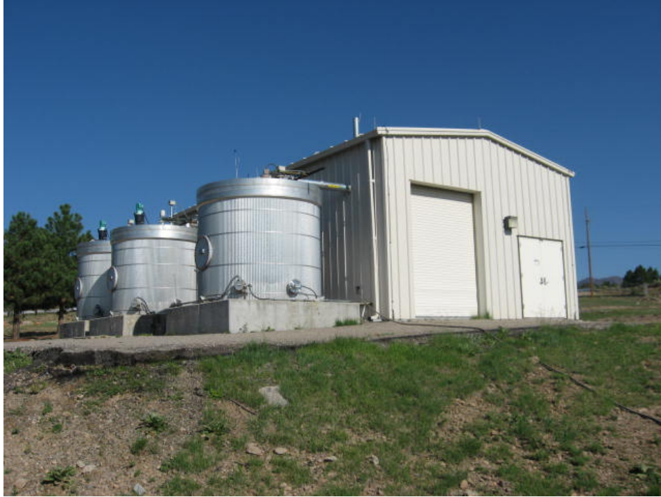
Photograph - NPDES-05A055-18-004 High Explosives Wastewater Treatment Facility (HEWTF)
