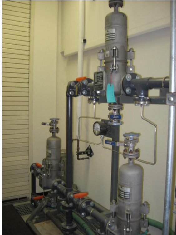
Photograph - NPDES-05A055-18-008 HEWTF - Cartridge Filters
